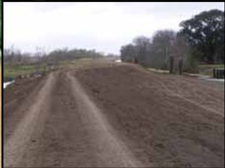
Levee Repairs in Valentine
