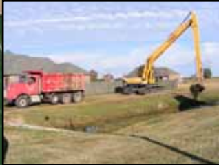
Rienzi & Rosedown Canal Maintenance
