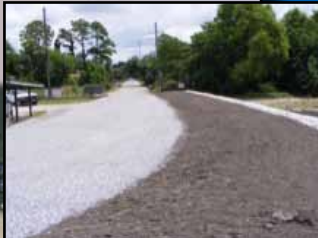
Levee Repairs in Larose
